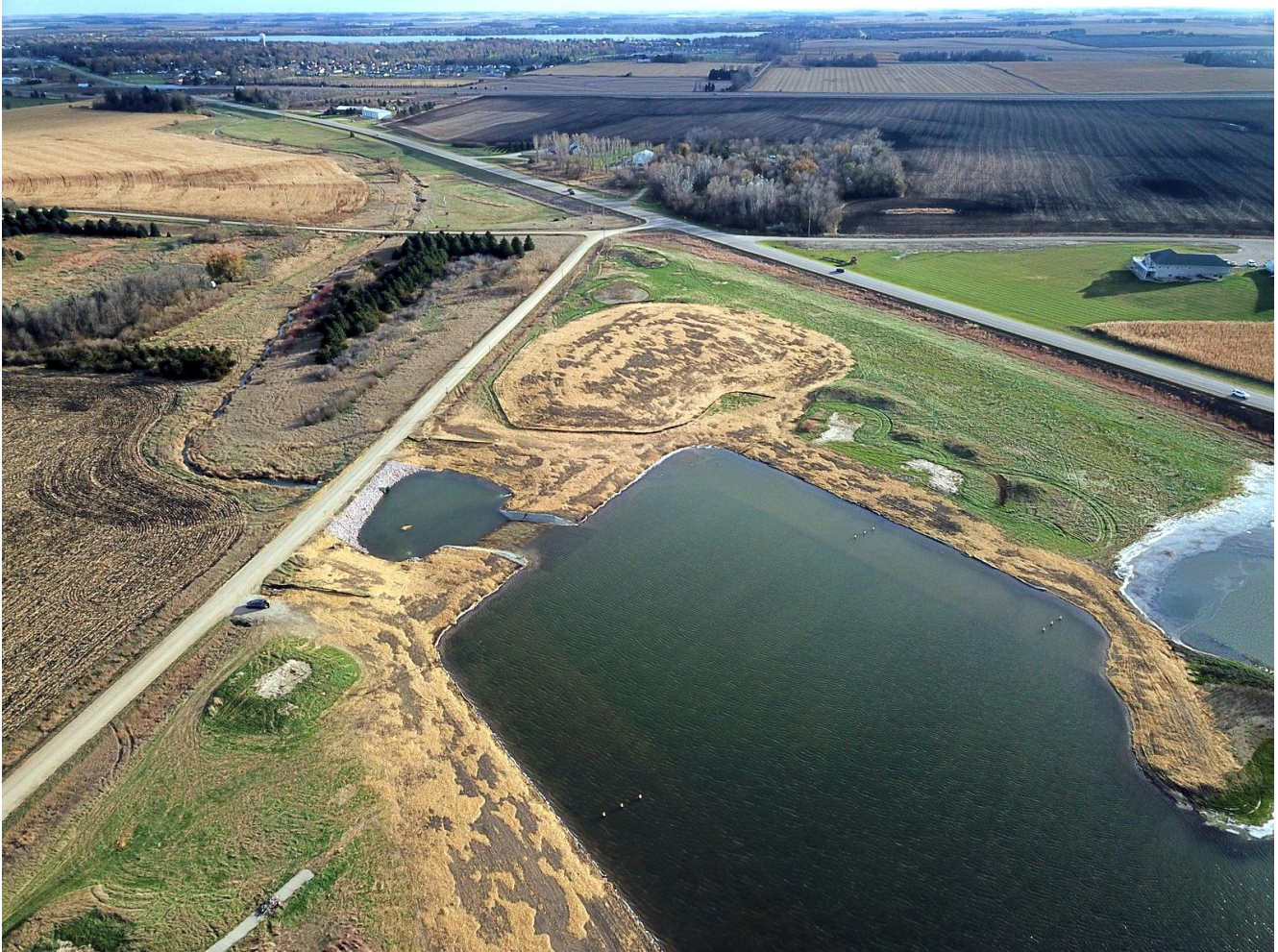
Construction underway at the Prairie View pond project site
