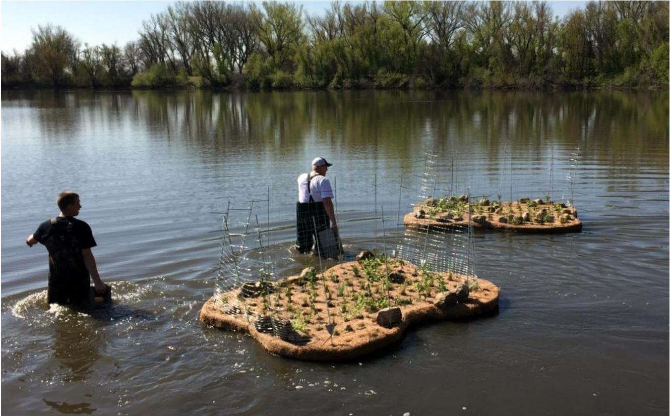
Installing Floating Island Wetlands in Sunset Bay
