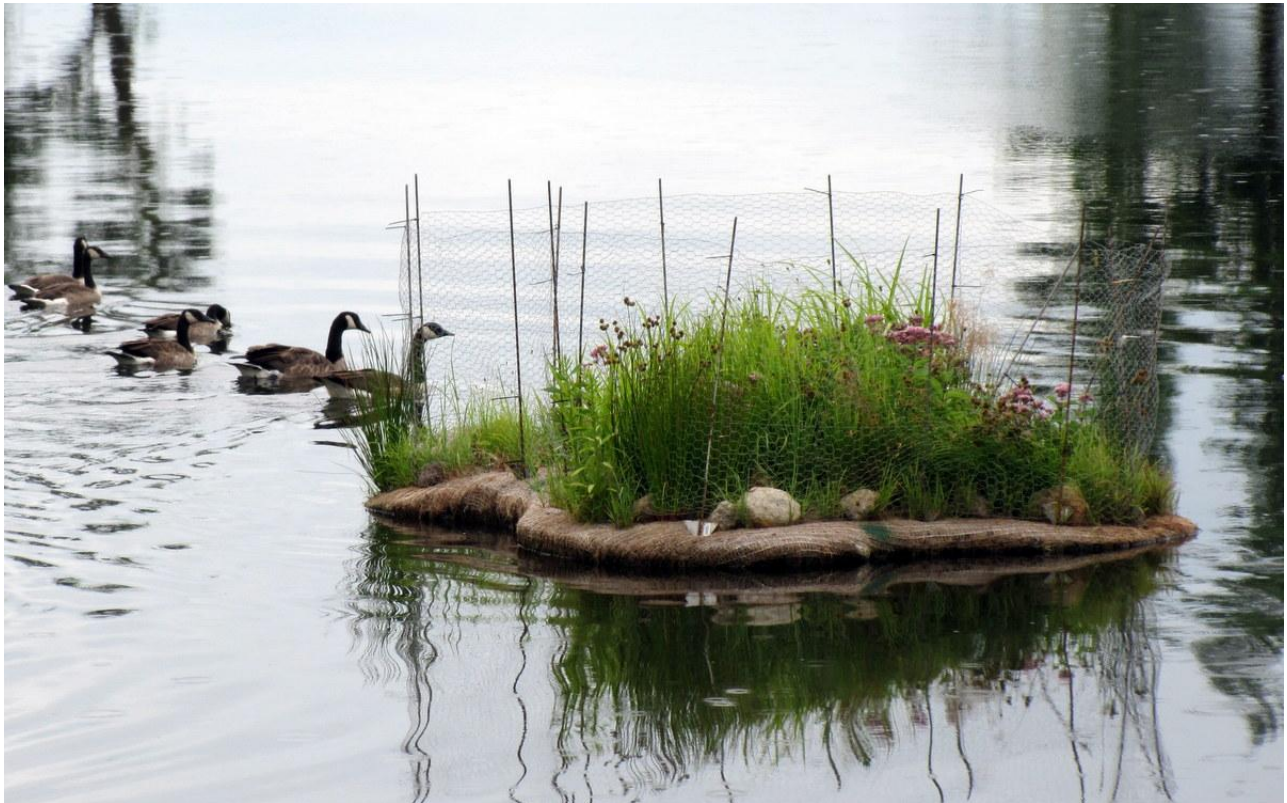
Floating Island Wetland at the Olson Regional Stormwater Pond
