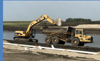
Sand filter benches installed in September.
