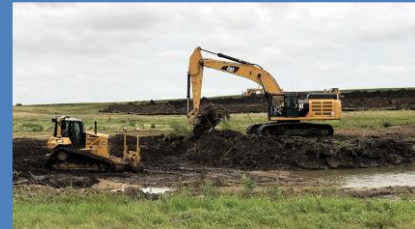
Construction begins in August.
