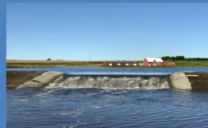
Emergency spillway completed a few days before October's big rain.
